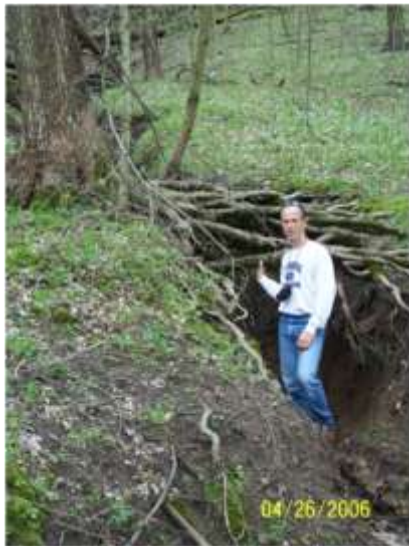
Ravine erosion in the bluffs of the Farm Creek Watershed
